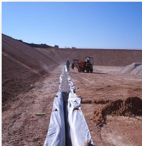
GEOTEXTIL, GRAVA TUBERIA GRAVA
